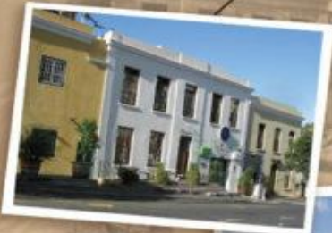
The entrance to Heritage Square
