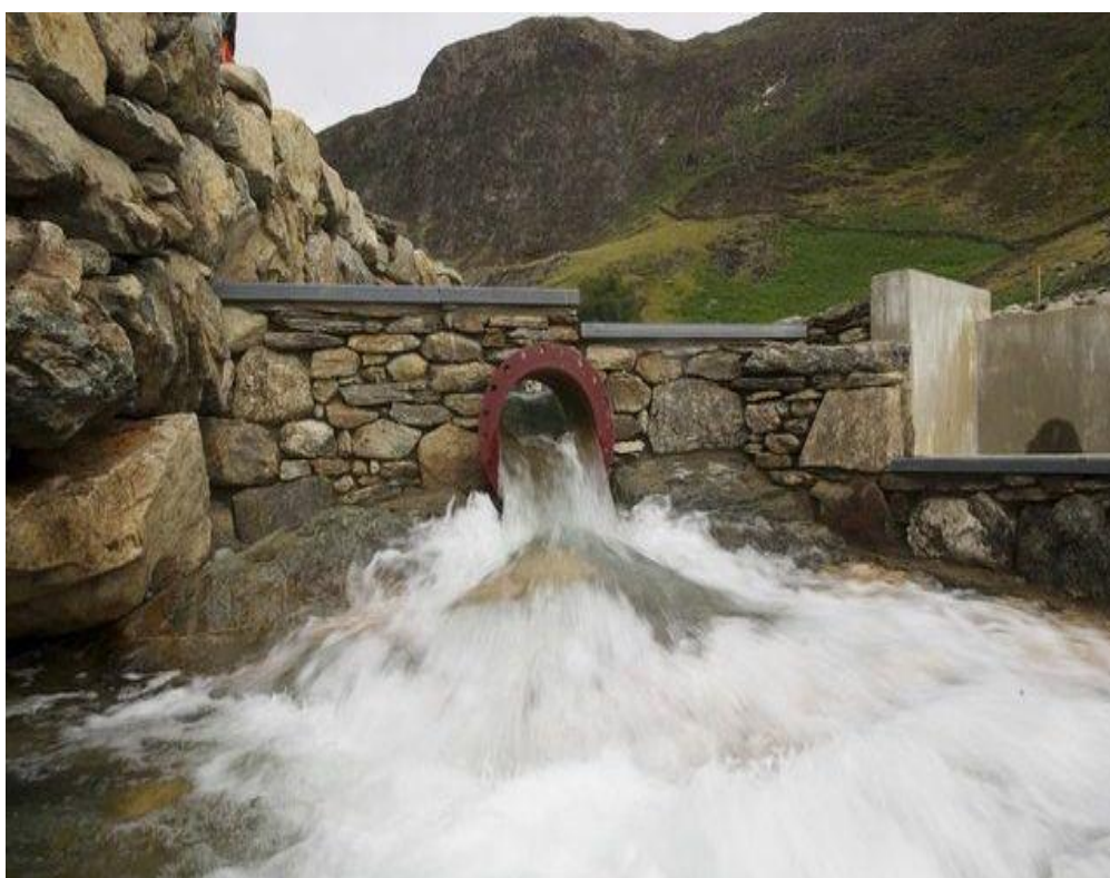
Energy Generation at Hafod y Llan (National Trust for England, Wales and Northern Ireland)
