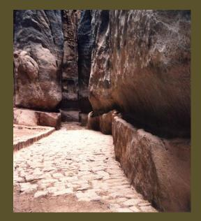
RESULT: Safe passage for tourists and reduction in damage to monuments due to flash floods (re-establishing the original breadth and slope of the Siq and construction and restoration of dams and related hydraulic features).
