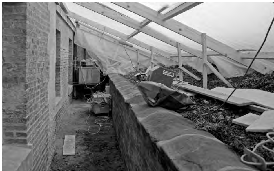
The north light well in its heated tent. © National Trust/John Moorey
