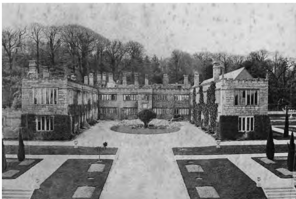
Lanhydrock House in April 1881, soon after the fire. Although the roof has been lost, the Jacobean walls remained intact. It took four years and an investment in excess of £100,000 to restore the house to its former glory using the latest in Victorian fire-proofing technologies. © National Trust/Lanhydrock
