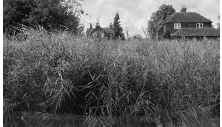
Bodiam Castle reed-bed sewage system in its first growing season (September 2011), with Castle Inn public house in background. © Chris Weedon
