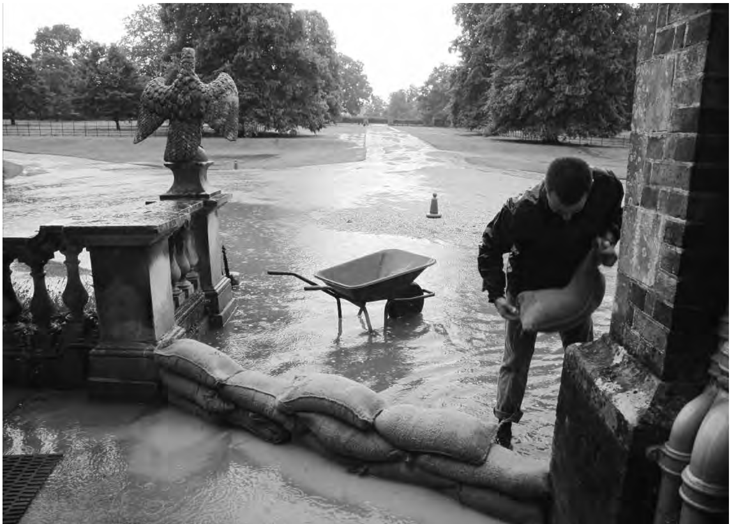
Building flood defences at The Vyne, Hampshire, as water from the overflowing lake rushes into the house, during the July 2007 flooding. © National Trust Images/John Hammond
