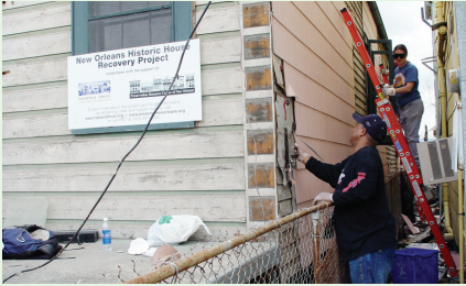
Repairing damage in New Orleans
