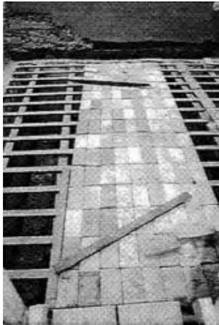
The reconstruction of the flat ceiling and roof utilizing recycled historic ausubo (bullet wood) roof beams, slats and brick in the Casa Ramón Power y Girth Restoration Project Old San Juan, PR (1994).
