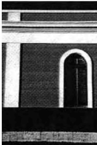
Detail of side facade showing final result of compatible finishes for plasters and lime washes. Lighthouse at Las Cabezas de San Juan in Fajardo, PR (1991).
