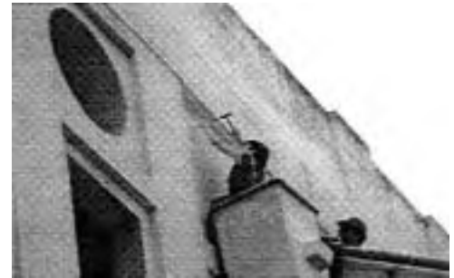
Ballajá Barracks material sampling from a high area of the building to assure least altered surfaces (1986). Done with the help of a "cherry picker" from the Electric Energy Authority
