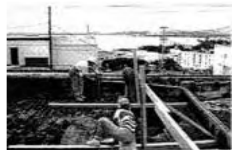
Inspection fieldwork in progress at Casa Ramón Power y Giralt in Old San Juan, PR (1992)
