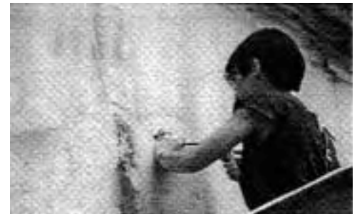
Ballajá Barracks material sampling from a high area of the building to assure least altered surfaces (1986). Done with the help of a "cherry picker" from the Electric Energy Authority
