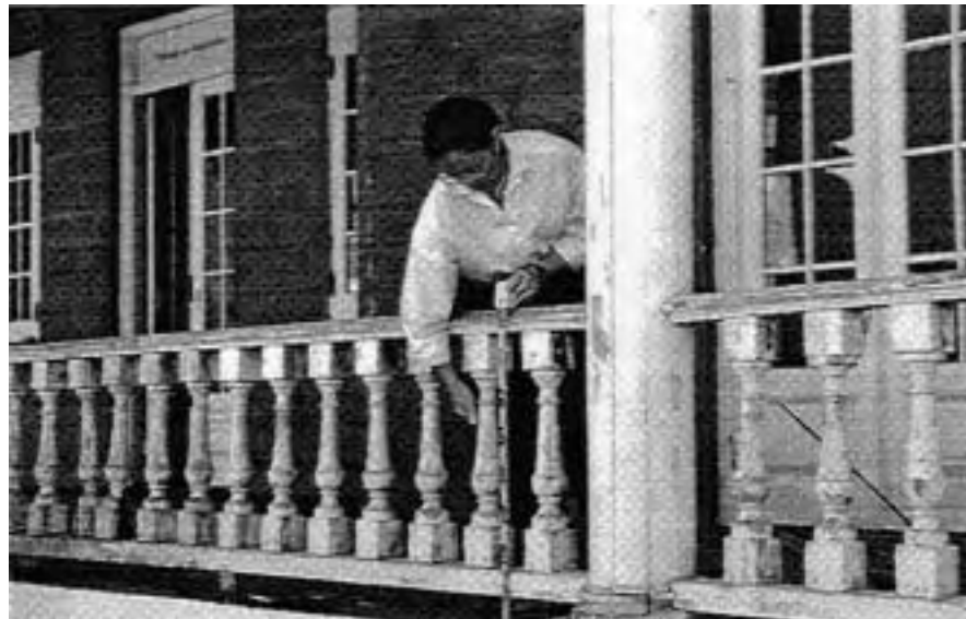
Colegio de Arquitectos Headquarters Inspection work (1993)
