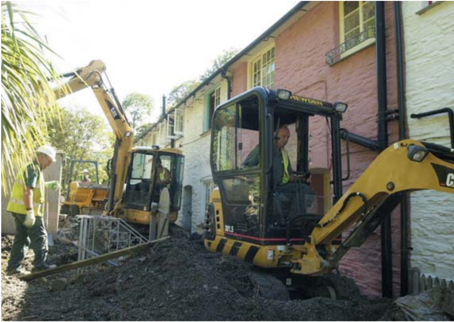
Environment Agency staff clear flood debris behind Marine Terrace in Boscastle
