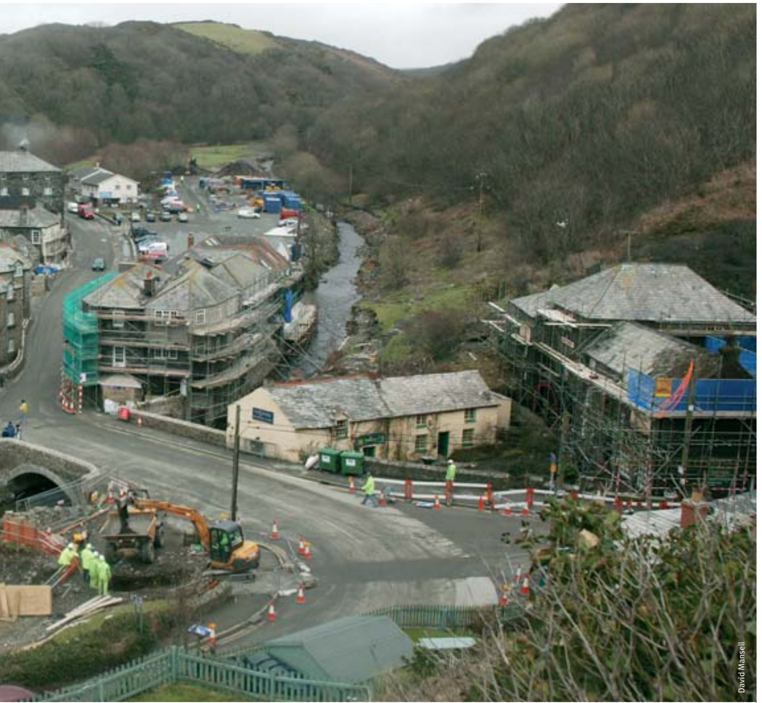
Regeneration: A new culvert is laid along side the Jordan as rebuilding work continues at Boscastle
