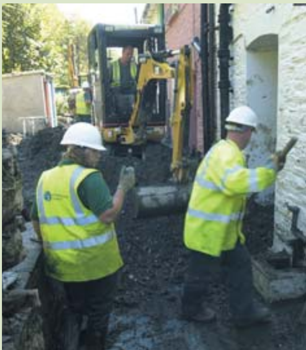
Environment Agency staff clear flood debris behind Marine Terrace in Boscastle
