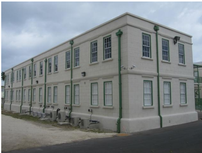
(Photo shows the South wing of the Nightingale Nurses Home building )
