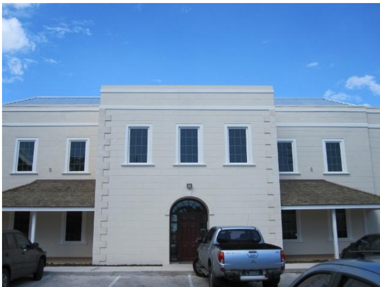
(Photo shows the South Entrance, with the new portico and verandah, and restored fenestration)
