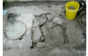
Bottom: 19th century outbuilding at Whitehall, area in white
