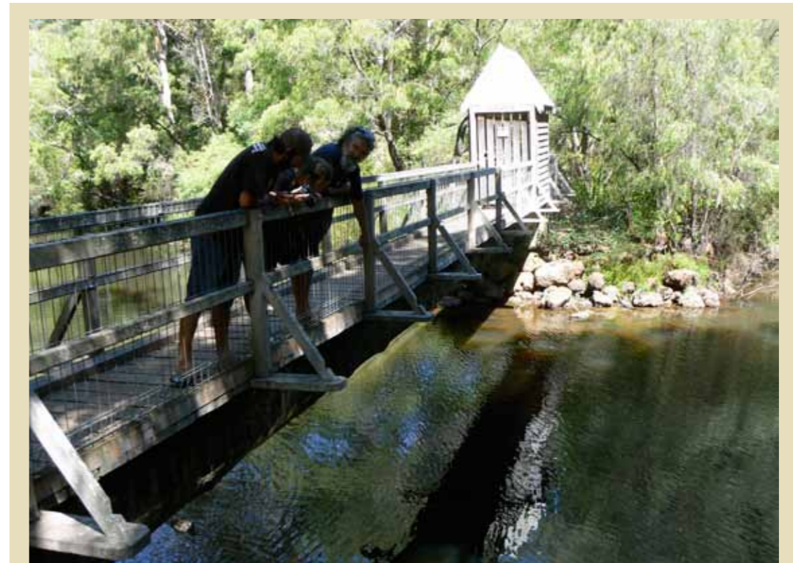
Assessing the condition of Wooditchup (the Margaret River), Rails Trails project. (Myles Mitchell, 2011)
