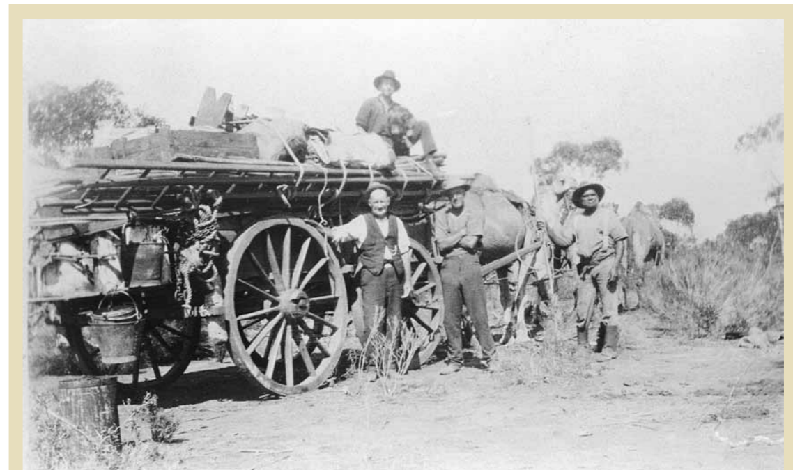
Aboriginal people worked along the pipeline including in maintenance gangs for the water supply scheme. This photo was taken in the 1930s near No 7 Pump Station (Gilgai). (R Birss nee Wall, c. 1930)
