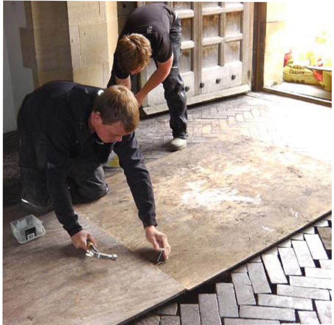
Above Installing the temporary floor
