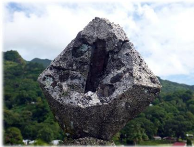
Damaged pinnacle due to corroded rebar.
