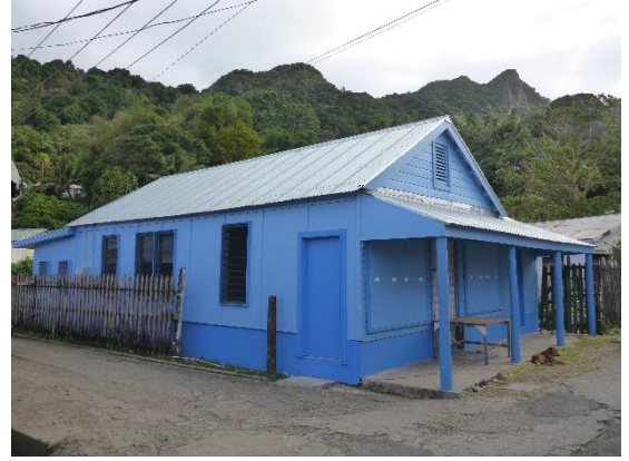
27-7-2014 Old front doors have been replaced
