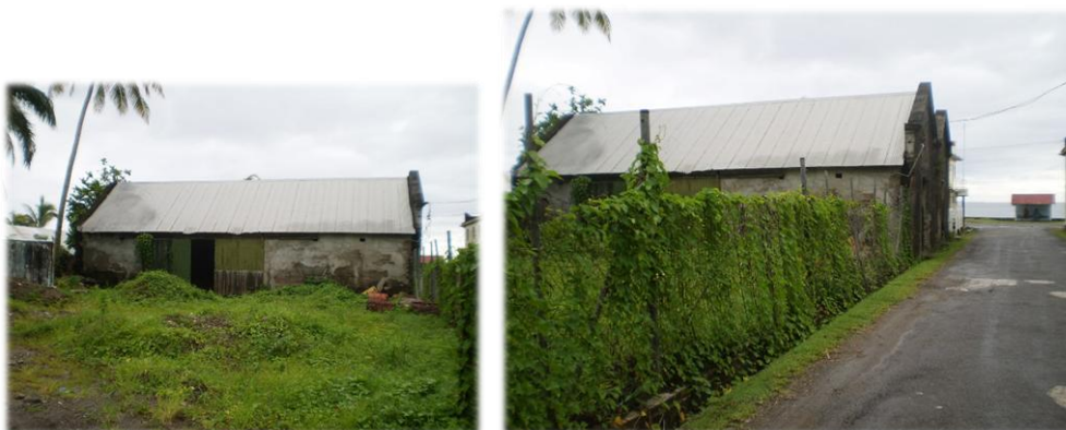
The west side of the stores c.2010.
