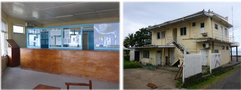
The building in December 2013 before renovation.
