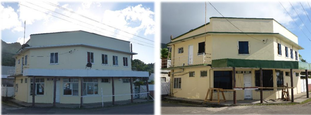
Start of the renovation in April 2014 by aluminum ones July 2014
