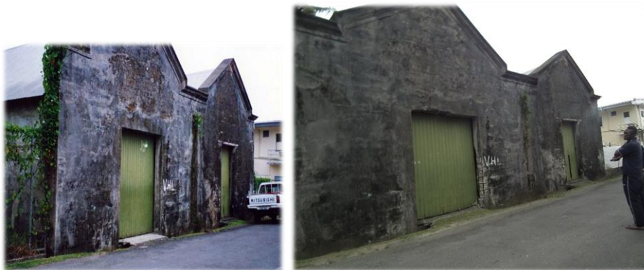
The stores still unpainted c. 2010
