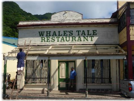
Renovation Veranda October 2014
