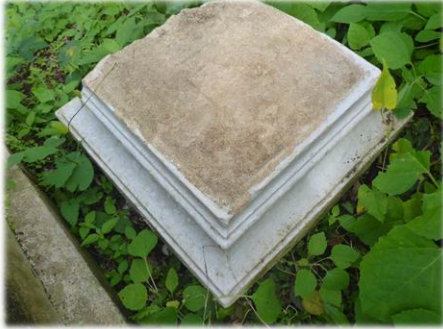
The Column cap upside down.
