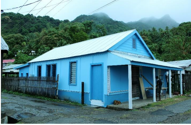
3-7-2014. Extra cement board has been added.
