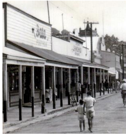
The building in 1956. The left top of the façade has been shortened
