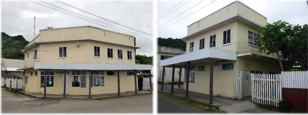
The building in December 2013 before renovation.
